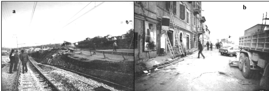
Fig. 1. Railway (a) and Flaminia Road (b) interrupted by the landslide.
