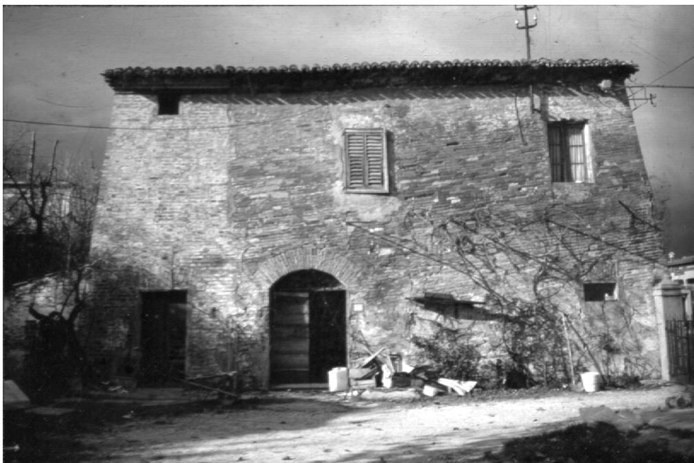
Fig. 7. The old postal-house sited on the T<sub>2</sub> trench. The house has undergone rotation, as can be recognized from the ancient repairs.
